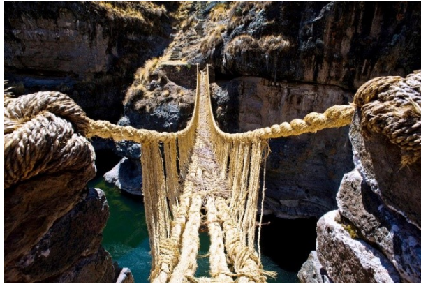
Fig. 5. «Q'eswachaka» – «an ancient rope bridge 28 meters long, connecting the banks of a canyon over the Apurimac River in Peru» (Житанська, 2021).
